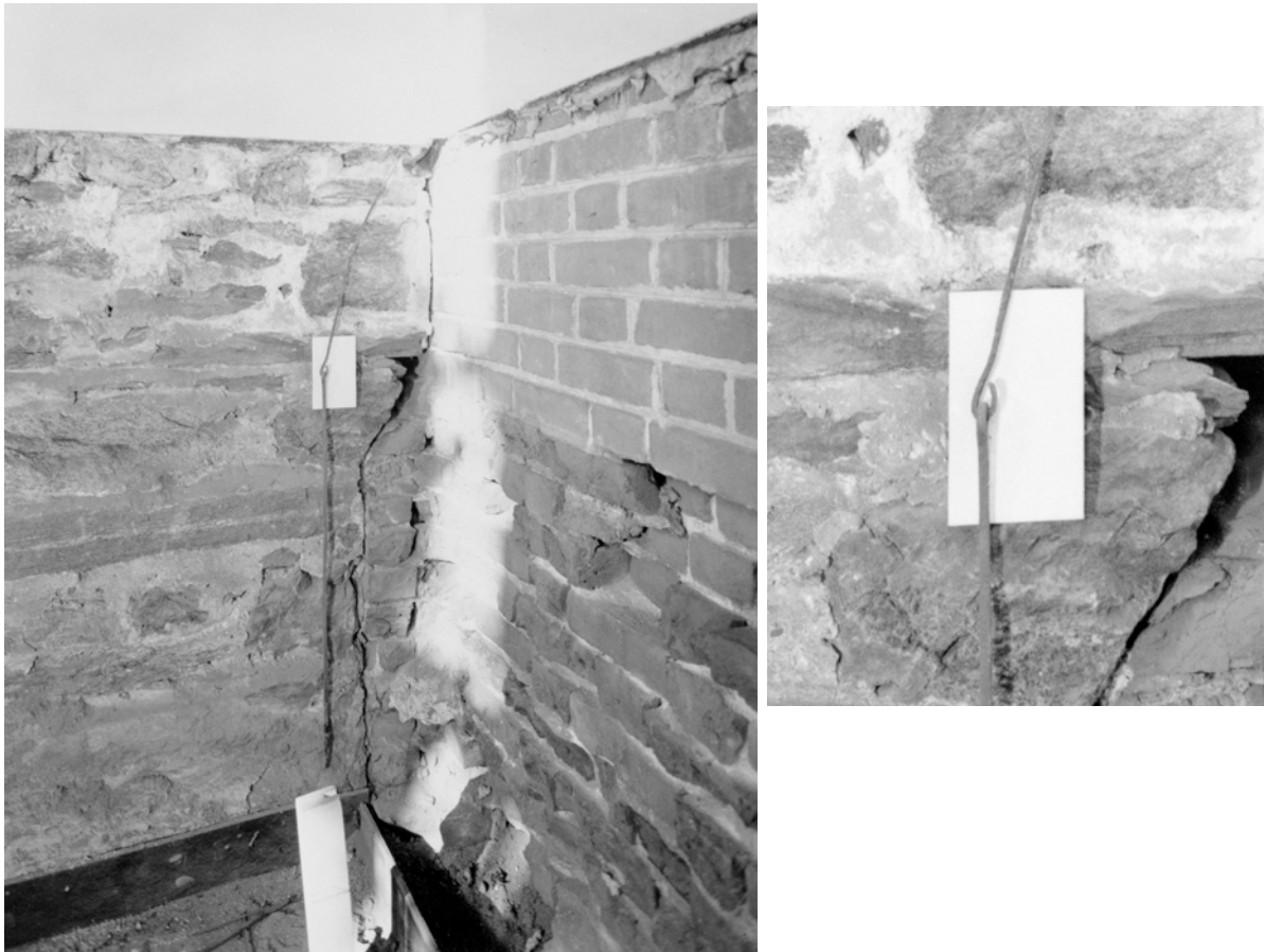
Fig. 3. Fragments of a down conductor, found under paneling and plaster on the inside wall of the northwest corner of the tower stairwell, on Independence Hall, Philadelphia. The inset on the right shows the hook connection in greater detail [Independence National Historical Park Collection].
